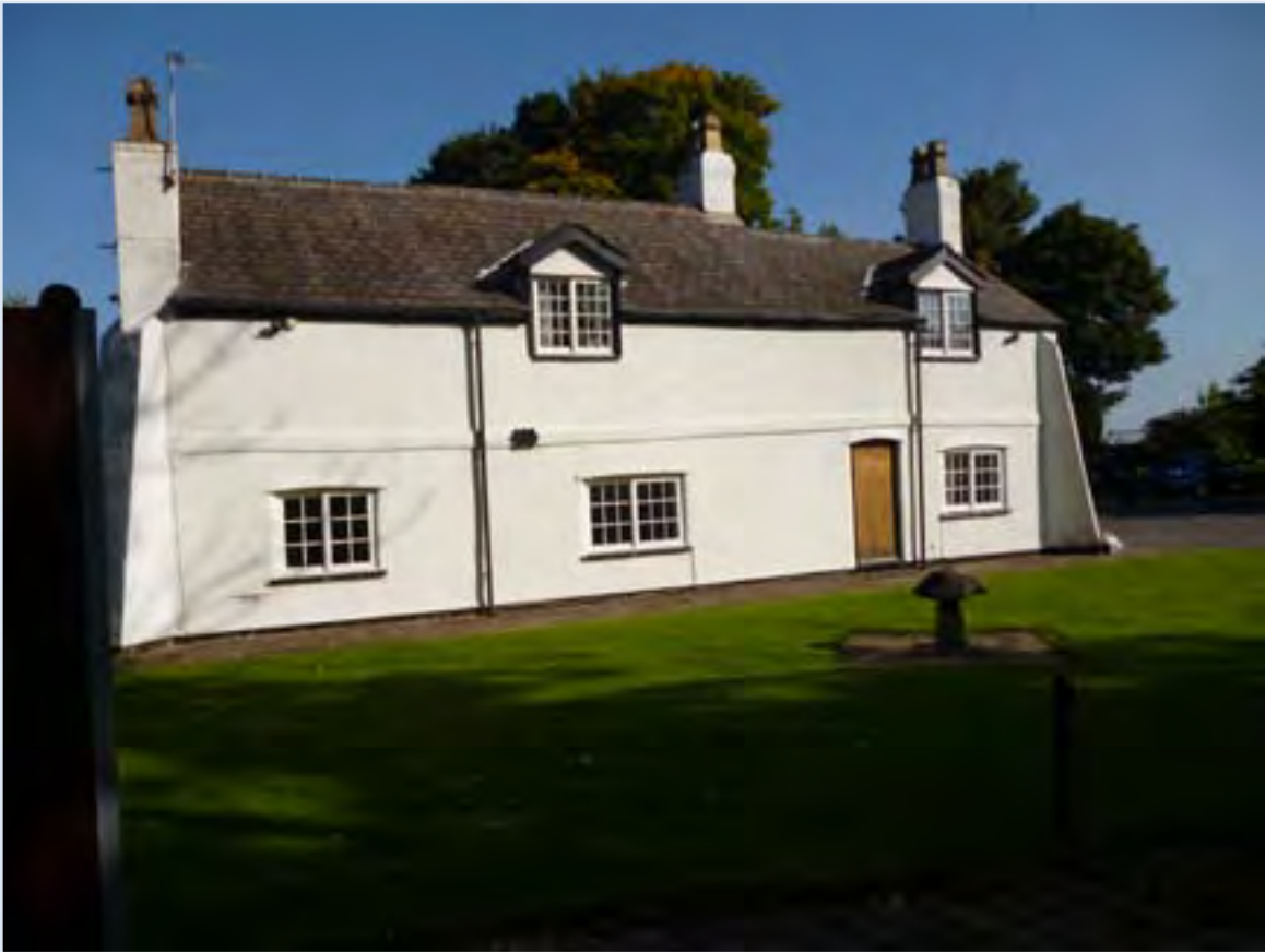
Plate MN 2.11- 4-East facing elevation of Formby House Farmhouse (Site 15)
