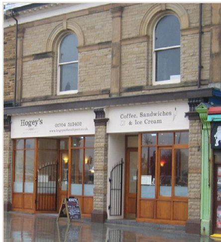
After work was completed
