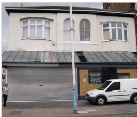
Before work began
