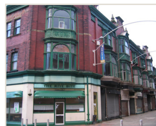
Before work began
