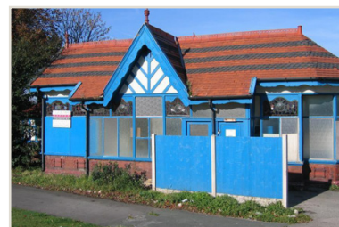
Vacant seafront building – before work
