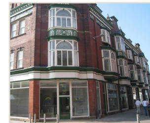
After work was completed
