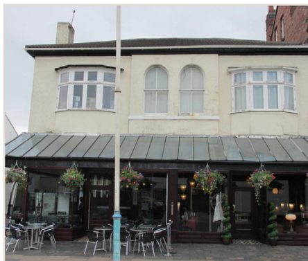
After work was completed
