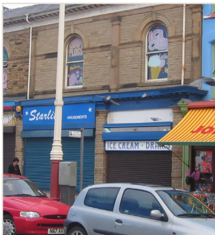
Before work began
