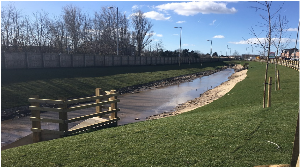
Swale (drainage system) – School Lane Poppyfields
