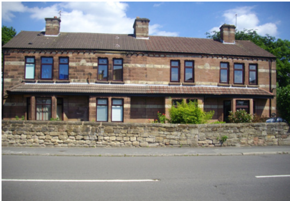
158 – 160 Liverpool Road South
