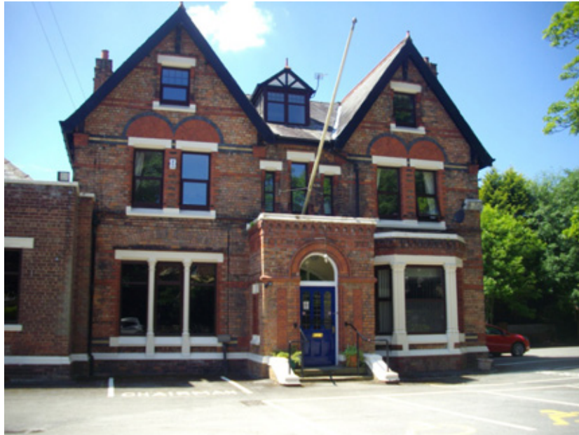
Kensington House, Station Road
