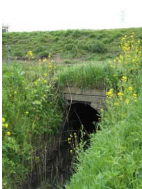
(v) Outfall pipe in south-eastern corner of site
