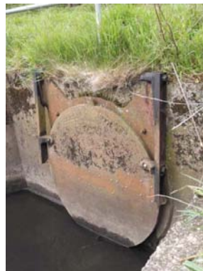
(vi) Flapped outfall to Downholland Brook
