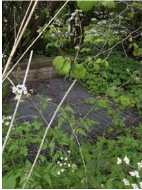
(i) Structure downstream of Formby Bypass
