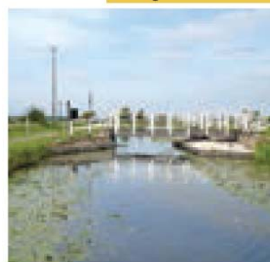
Holmes Swing Bridge
