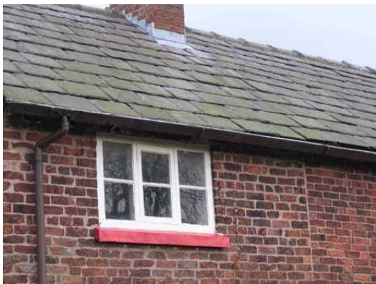
Casement Window at Lunt House Farm
