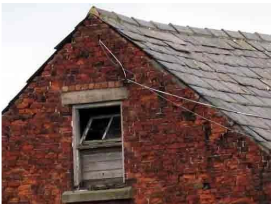
Slate roof on agricultural building at Rose Farm
