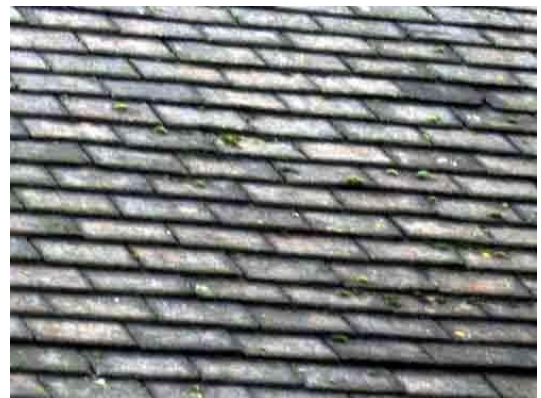
Original roof tiles on 1950s Estate
