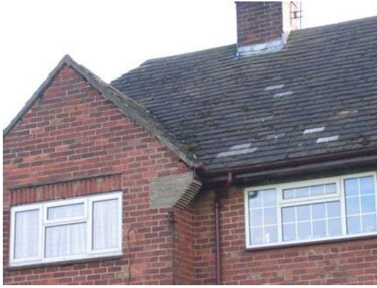
Windows in 1950s estate
