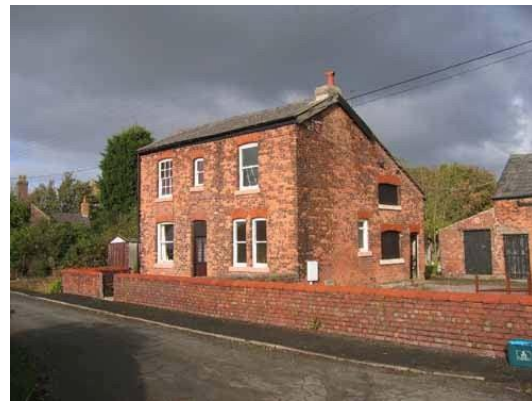
Vertical sliding sash windows at Rose Cottage
