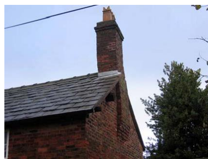
Chimney at Lunt House Farm
