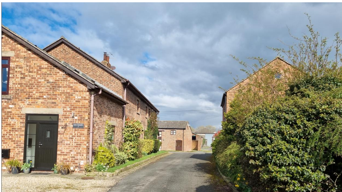
Kiln Barn, Hare Barn and Rigmaiden Barn viewed from Hall Lane looking north
