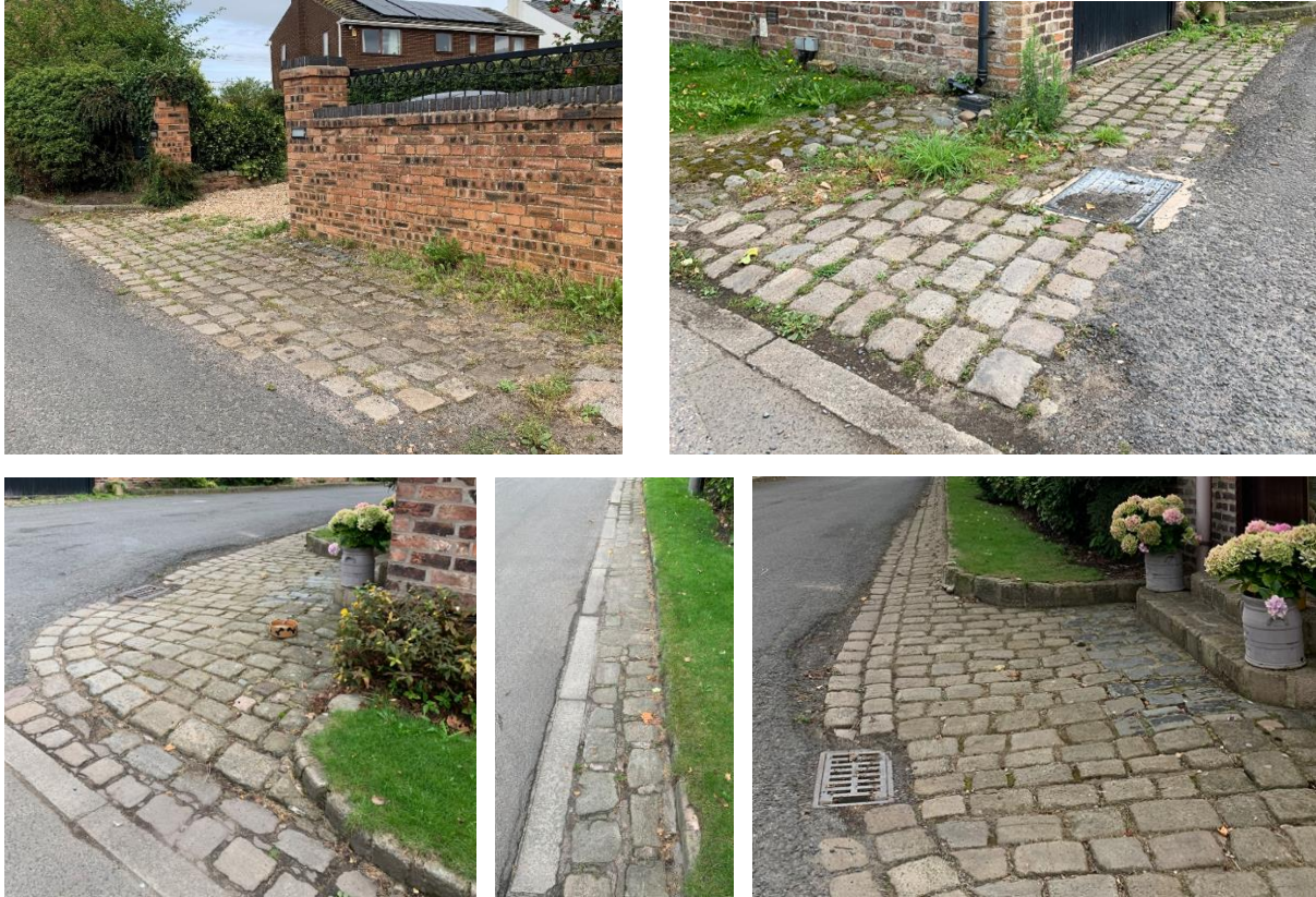
Examples of original cobbles in the floor of Carr Houses Conservation Area
