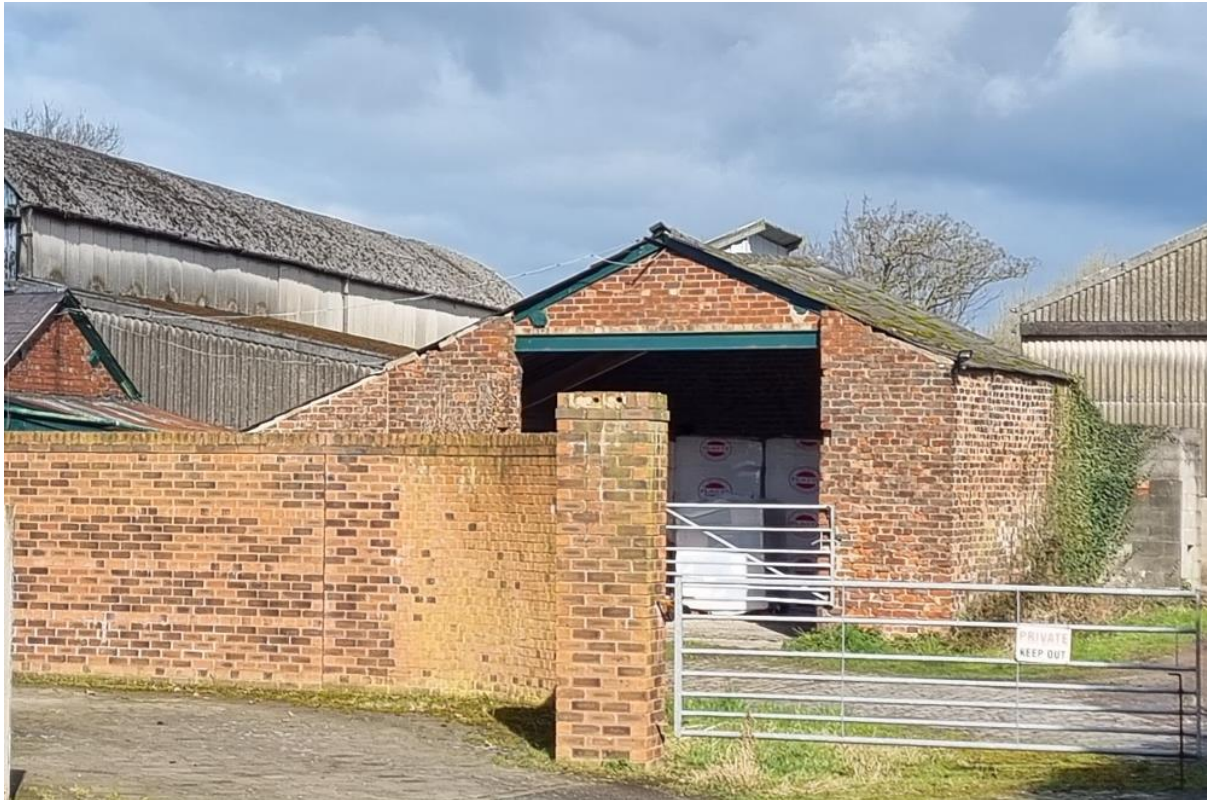
Square brick outbuilding associated with Rigmaiden's Farm
