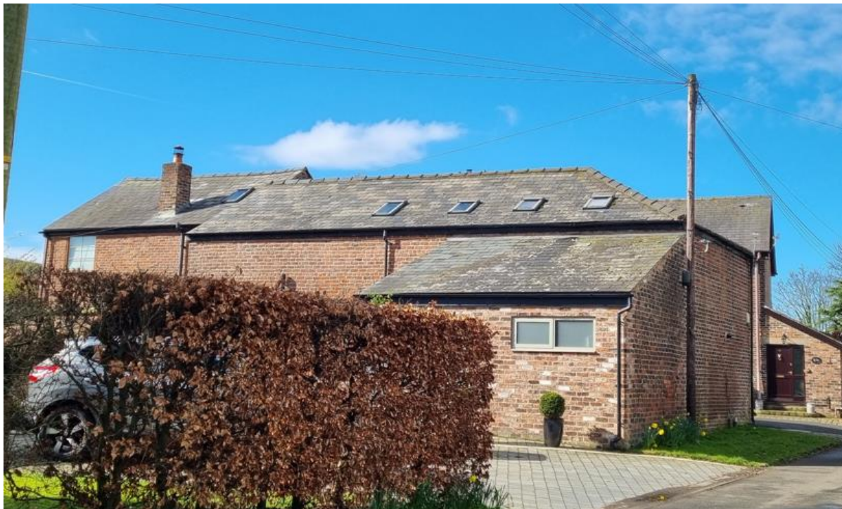
Roof lights at Hare Barn
