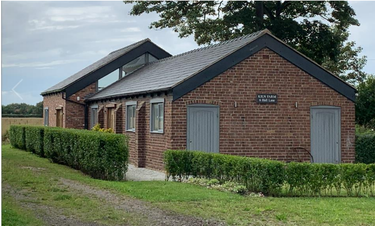
6 Hall Lane as an example of a sympathetic agricultural building conversion
