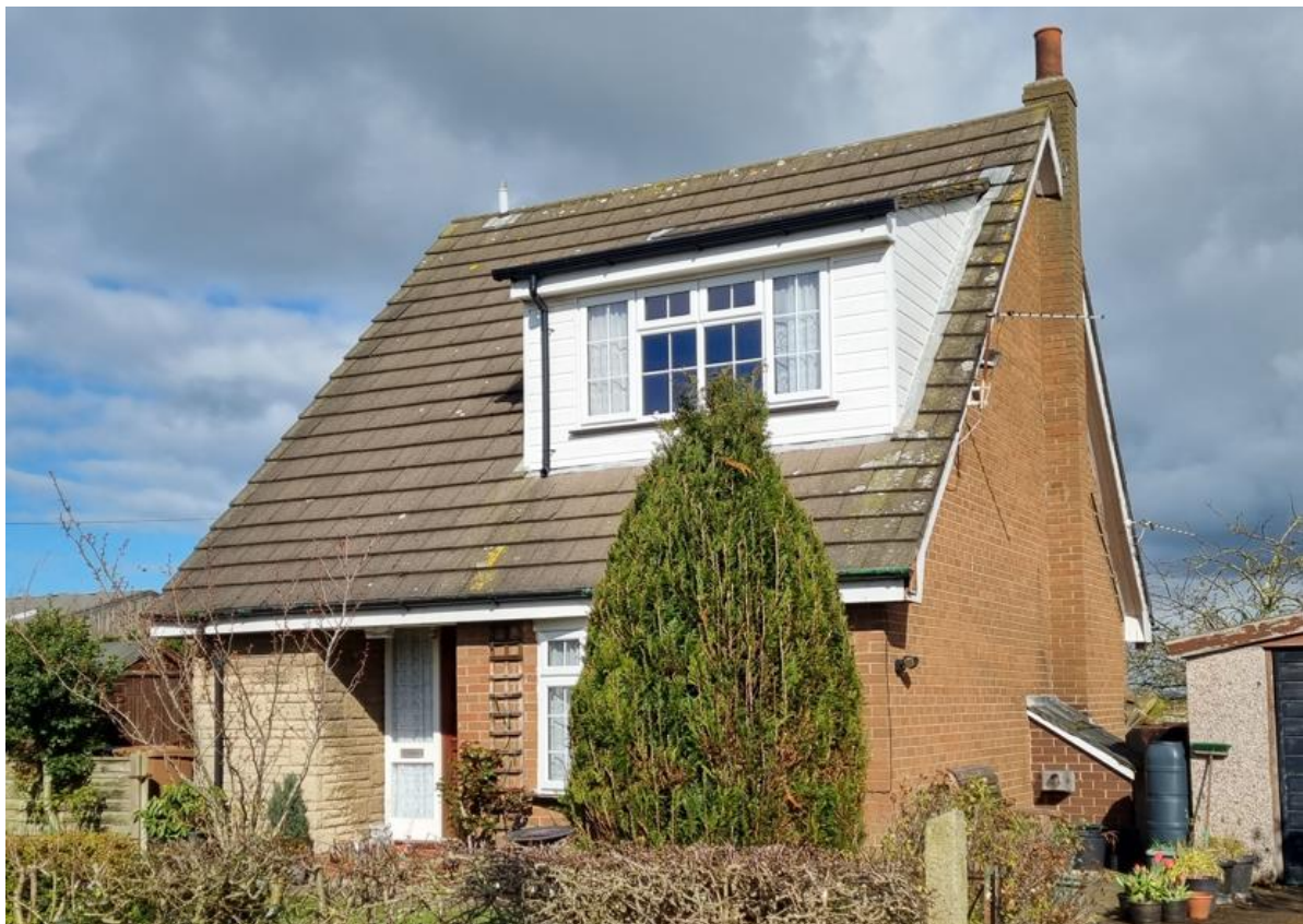
Roof at 111 Carr House Lane
