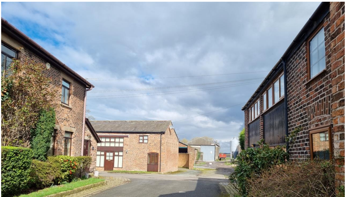
A view of the focal group of three barns, Kiln Barn (left), Rigmaiden Barn (middle) and Hare Barn (right) from Hall Land towards Carr Houses Lane
