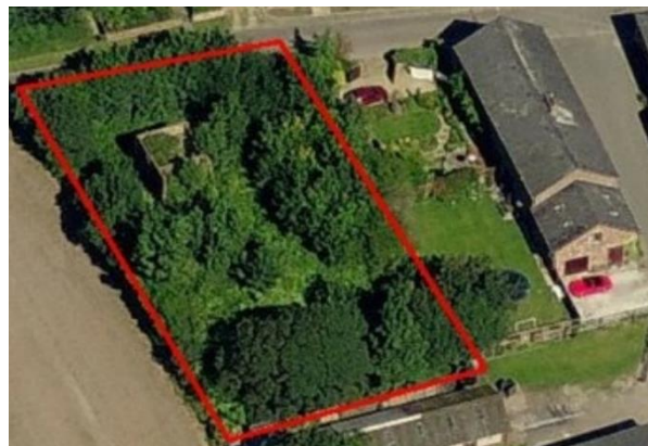
2014 Aerial photograph showing partial ruins of Kiln Farm farmhouse (since demolished)
