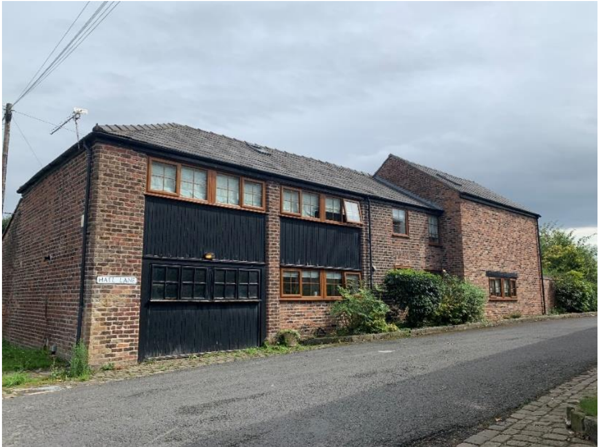
Gable roof at Hare Barn
