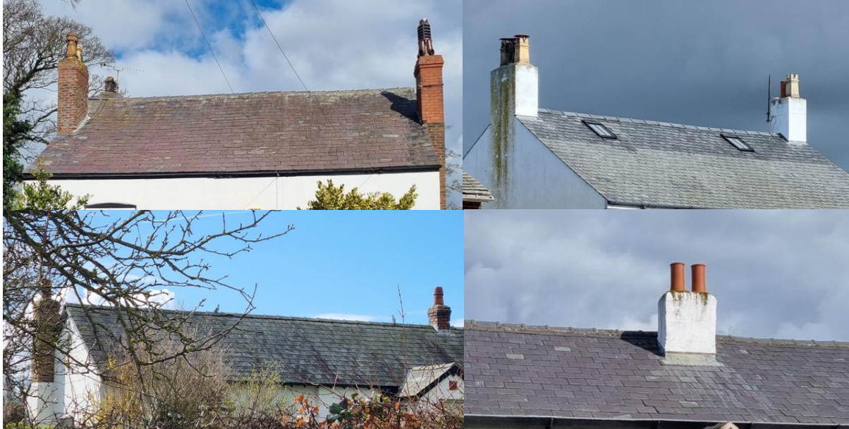
Chimneys within Carr Houses Conservation Area
