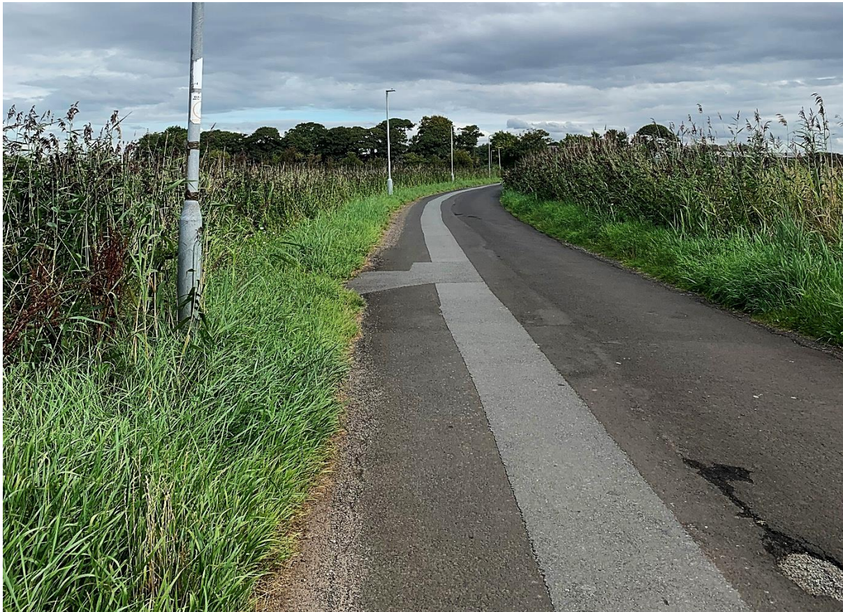
View A – Carr House Lane (West)
