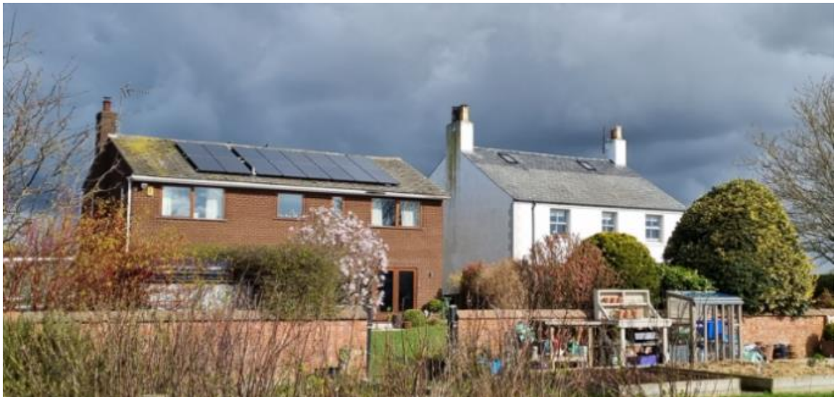
View of 122 and 124 Carr House lane viewed from Hall Lane showing the choice of design for the 20 th century house at Number 122 to create a harmonious roofscape with the traditional buildings
